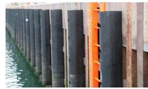
• To perform as bumper to protect the hull and bearing facility from damages
